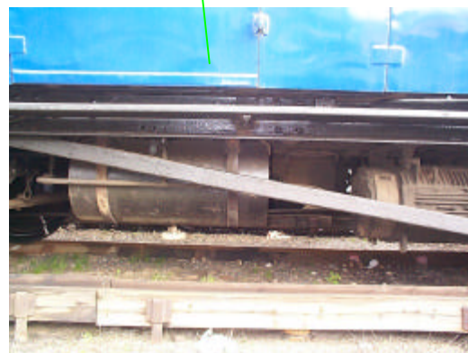
Main Air Reservoir
