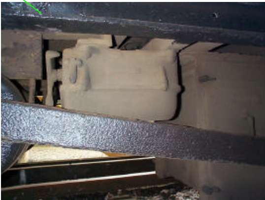
Main Power Switch
