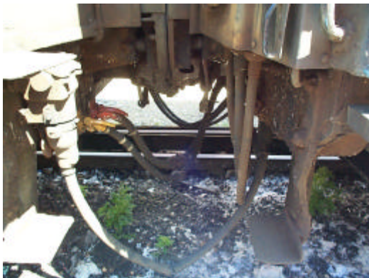
Jumpers connecting to DTC (right) (power side)
