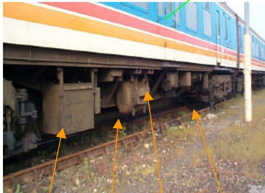
Battery Box, fuse box, MG resistor, MG set
