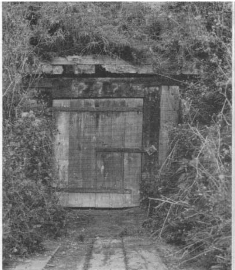
The railway drainage heading, kept securely bolted, which leads into the half-mile-long test tunnel which was bored in 1881 by the Beaumont machine
