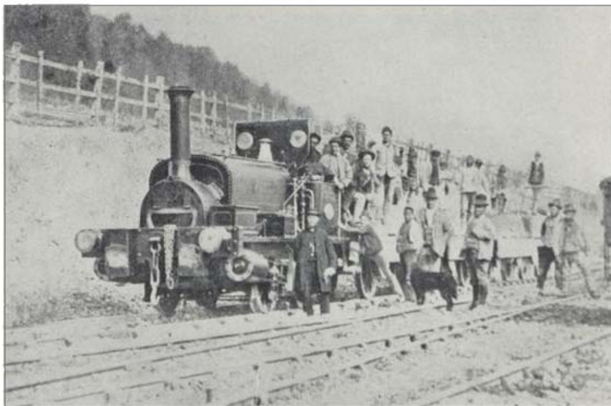
A photograph taken at Singleton in 1880, showing a construction train on the Chichester and Midhurst line, L.B.S.C.R., hauled by the Contractor's engine "Fred"
