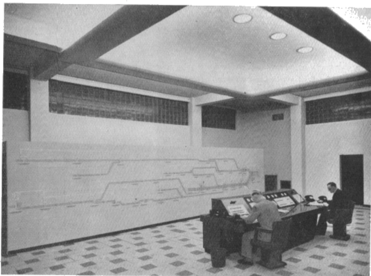
Mimic diagram and operators' desk at Raynes Park
