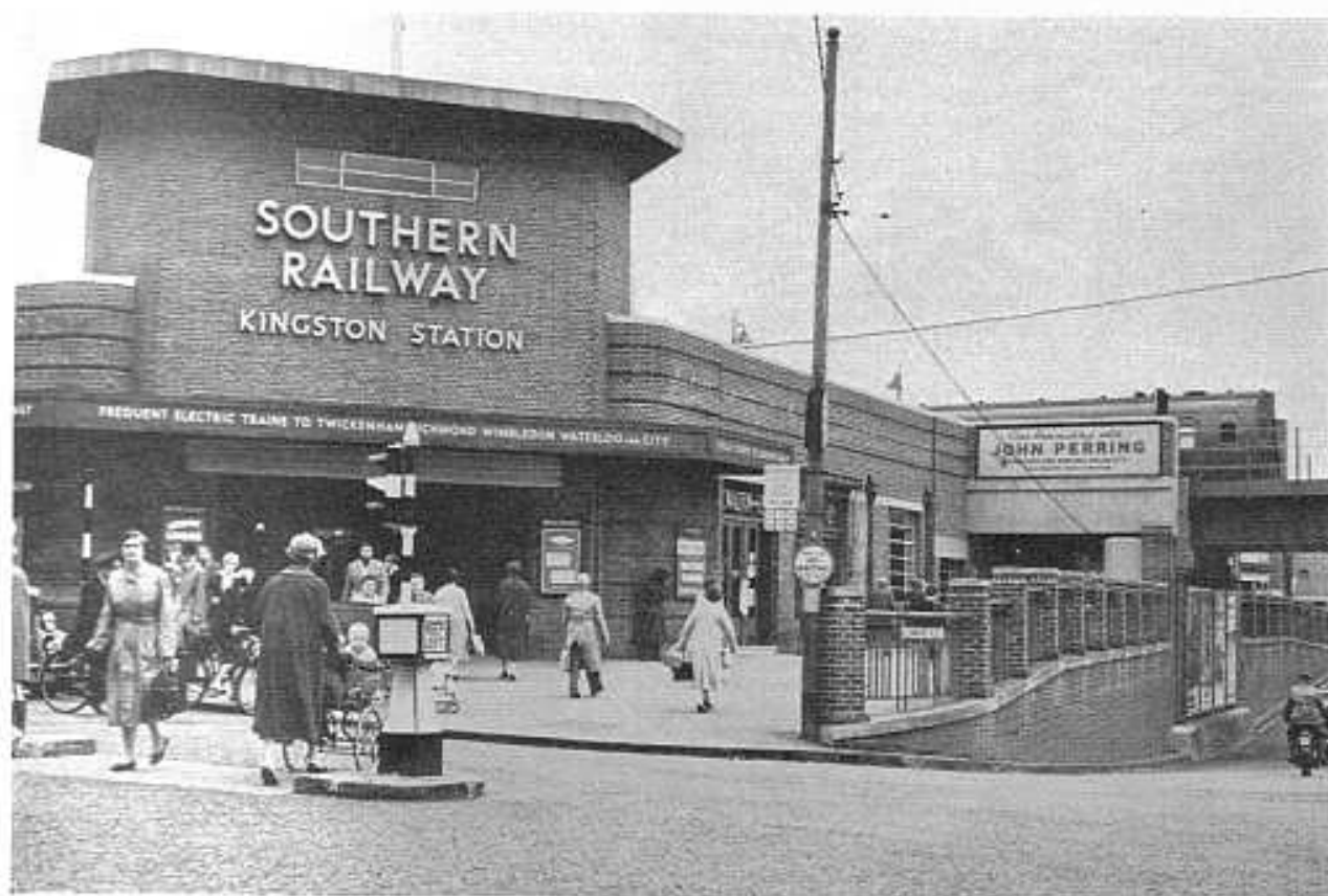
Exterior of the present station at Kingston
