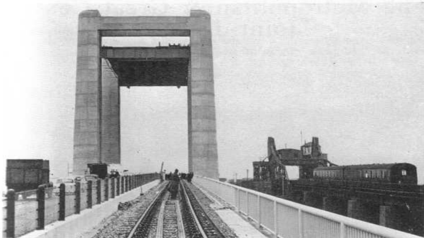
Lifting span of the new bridge in the raised position, showing the rail approach and a train crossing the old bridge
