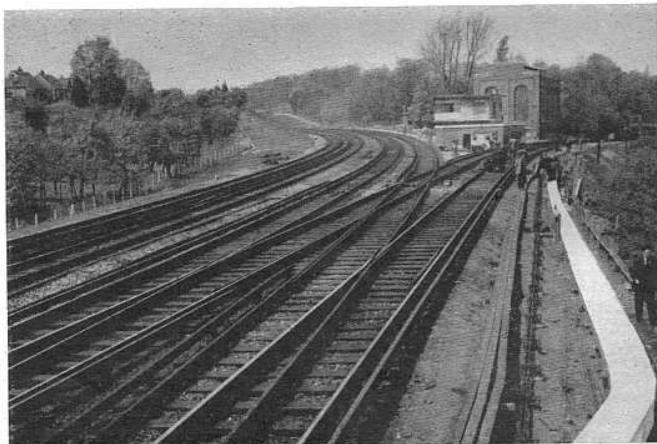
New junction at Shortlands, with the Catford Loop (on the right), laid on September 6-7, 1958
