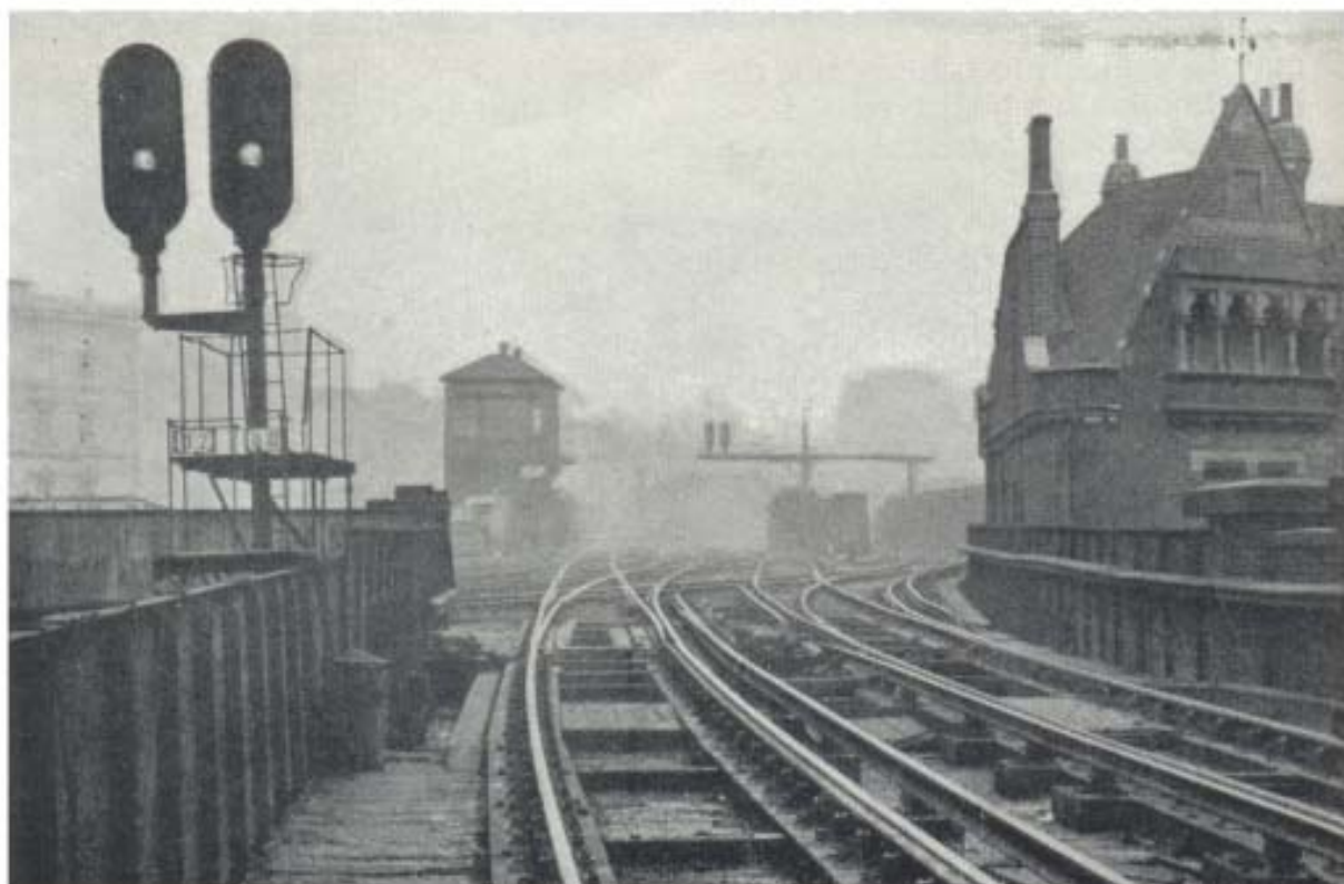
Looking towards Borough Market Junction Signal Box from the Charing Cross line
