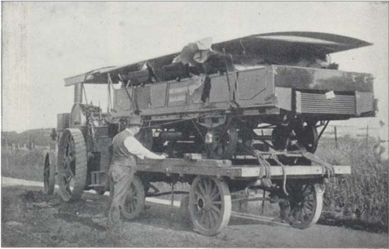
Drewry railcar, partly dismantled, being transported by road in course of delivery to the F.Y.N.R.
