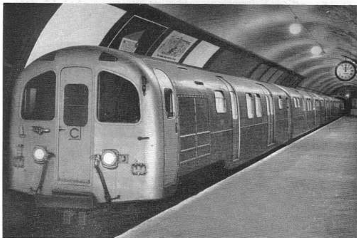
Recent view at Bank Station showing a train of the all-steel stock which replaced the original equipment in October, 1940
