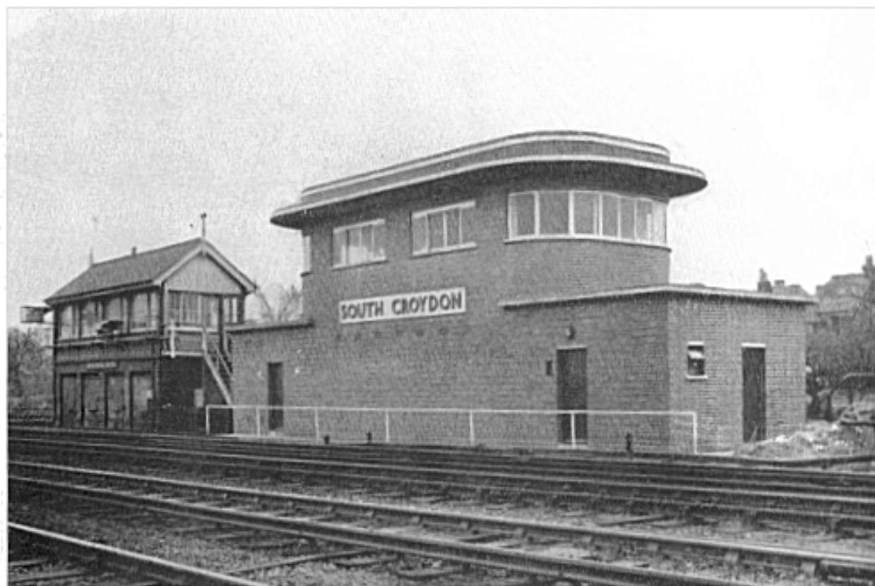
The new signalbox at South Croydon, with the old South Croydon Junction box, one of the two it has replaced on the left
