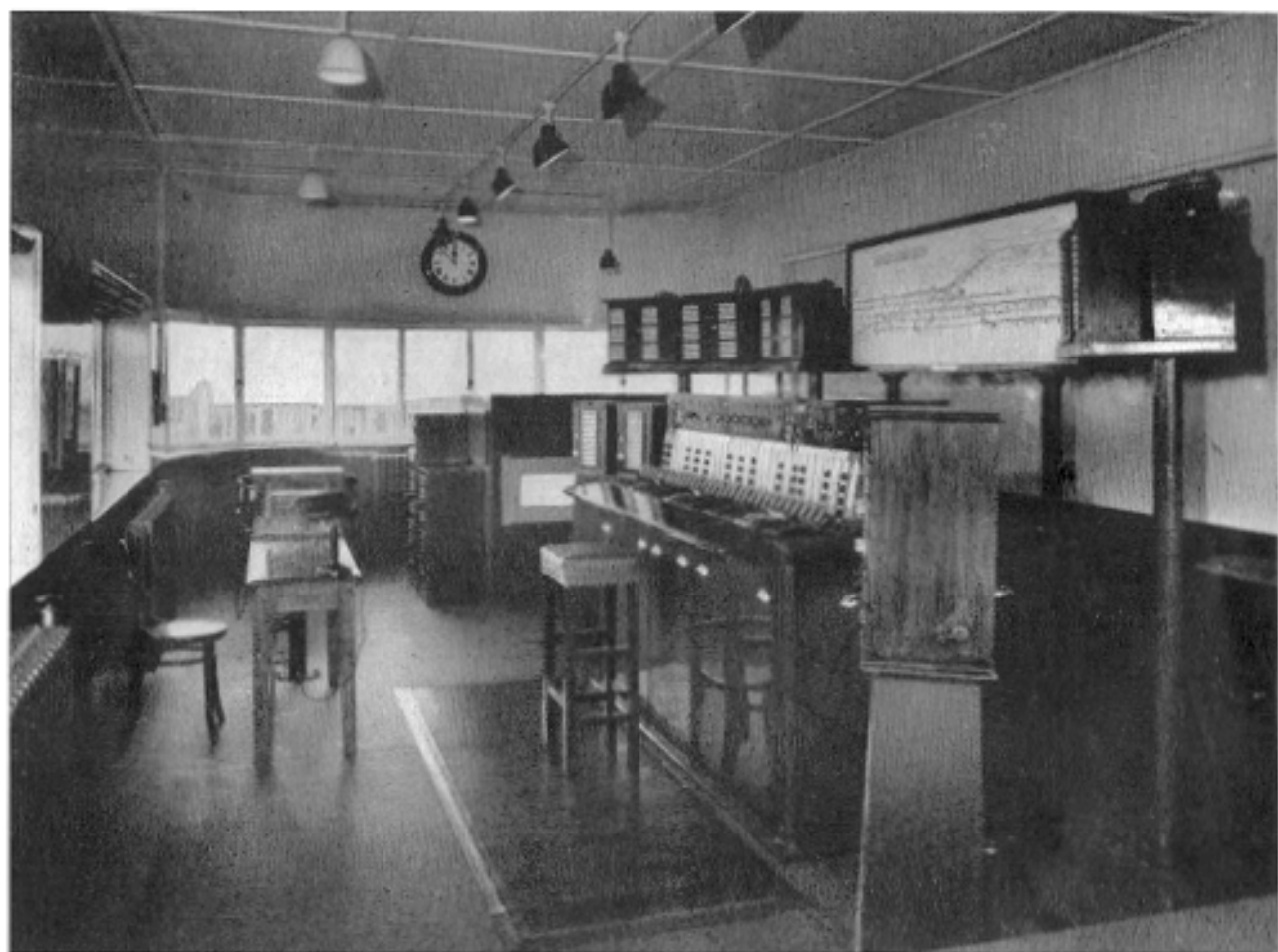
Interior of the new signalbox at South Croydon, showing the 31-lever frame and illuminated diagram
