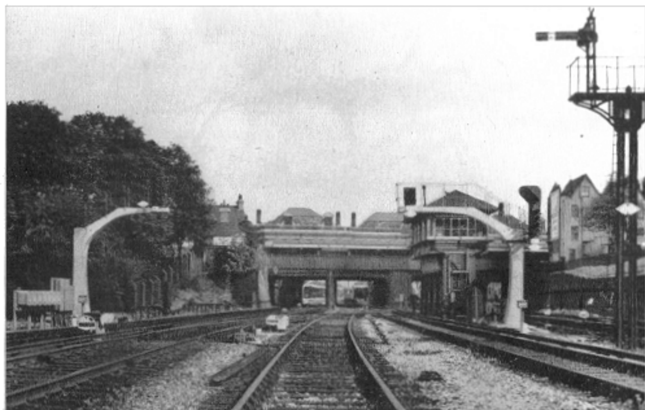
The approach to East Croydon Station from the south, shortly before the changeover, with new colour-light signals on concrete cantilevers
