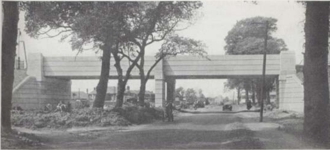
Double-span bridge over Ewell Road
